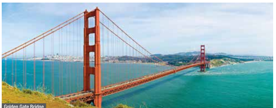
Golden Gate Bridge
